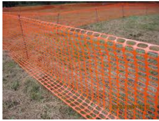
Fencing protects areas from compaction
