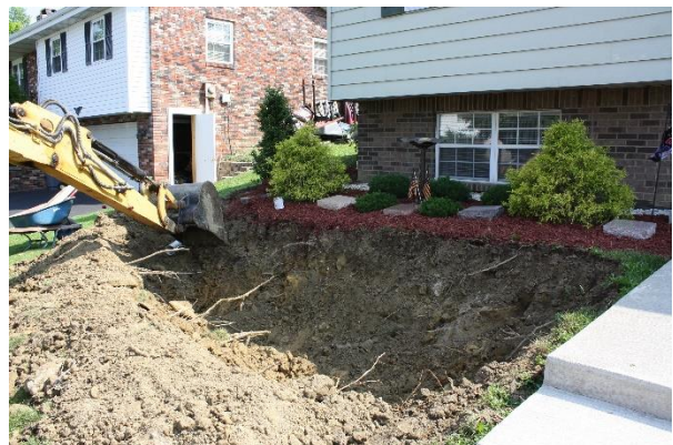
Excavate rain garden at least 10' from foundation
