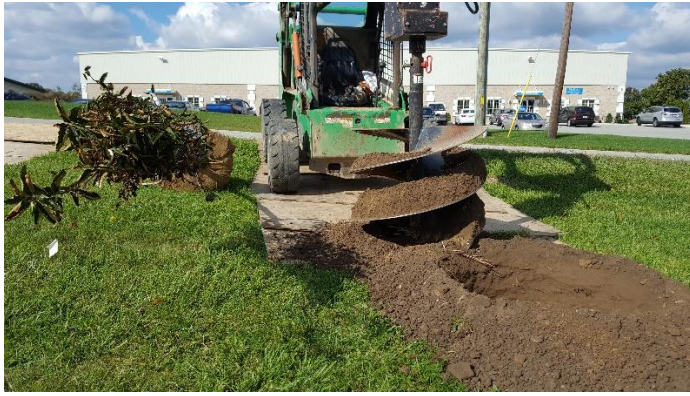
Plywood sheets protect lawn from compaction
