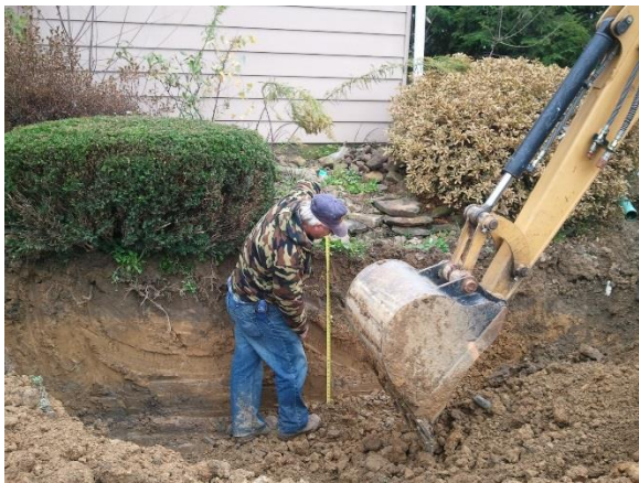
Excavate a drywell at least 10' from foundation
